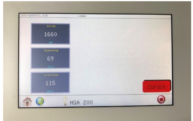
Lamp status monitoring
